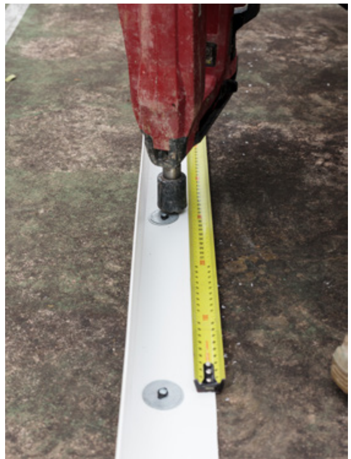
5: Fix angles to concrete slab through any of the following methods:
