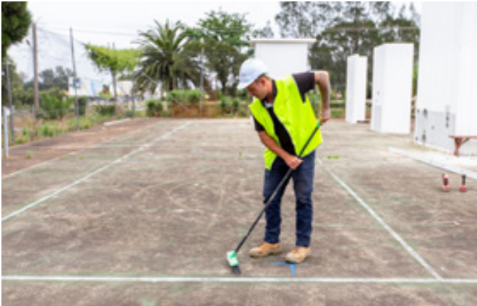
1: Clean substrate ready for set out.
