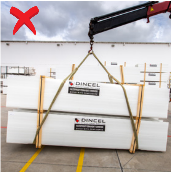
INCORRECT LIFTING (No lifting/spreader bar used)
